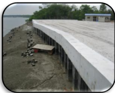
Rajah 2.2(a) Steel Sheet Pile Wall
