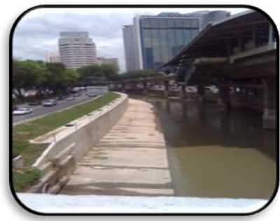
Rajah 2.2(c) Concrete Wall
