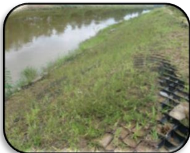
Rajah 2.2(d) Concrete filled Lining
