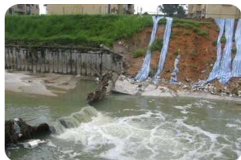
Rajah 2.3(i) Runtuhan Tebing di hilir Tebing
