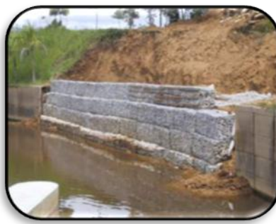
Rajah 2.2(b) Gabions Wall
